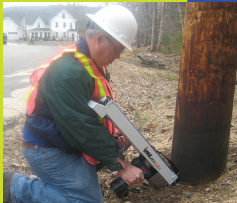
Figure 1. Inspecting Below Ground Level
